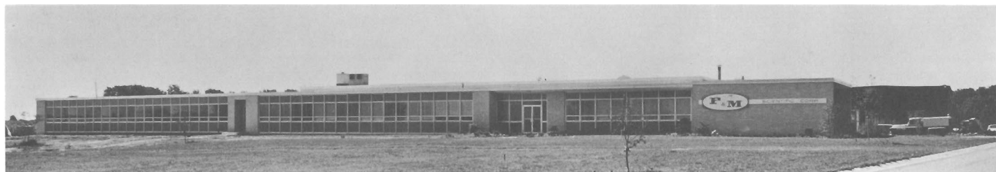
F&M's manufacturing facilities are located in this modern, low profile building.
